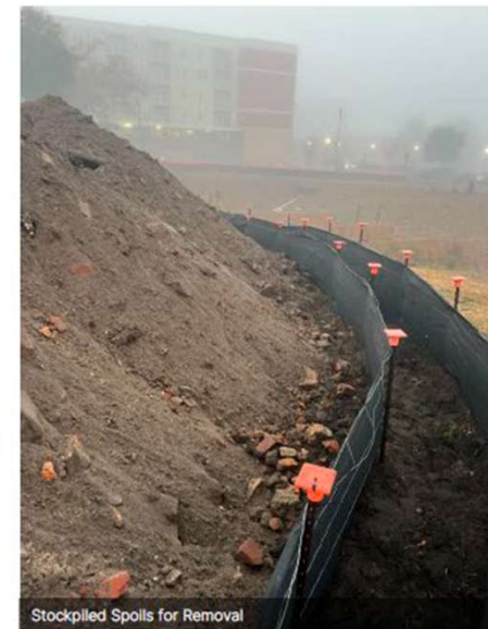
Stockpiled Spoils for Removal
