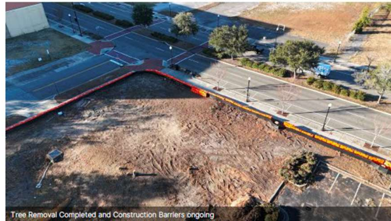
Tree Removal Completed and Construction Barriers ongoing
