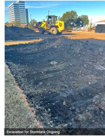
Excavation for Stormtank Ongoing
