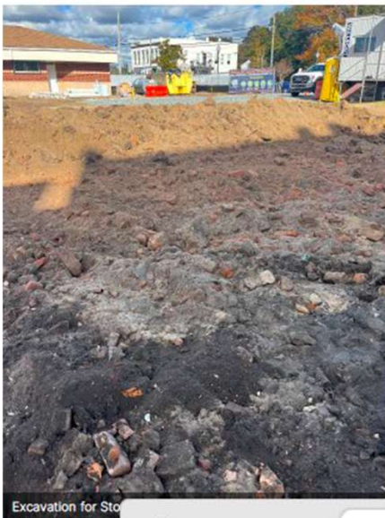
Excavation for Sto
